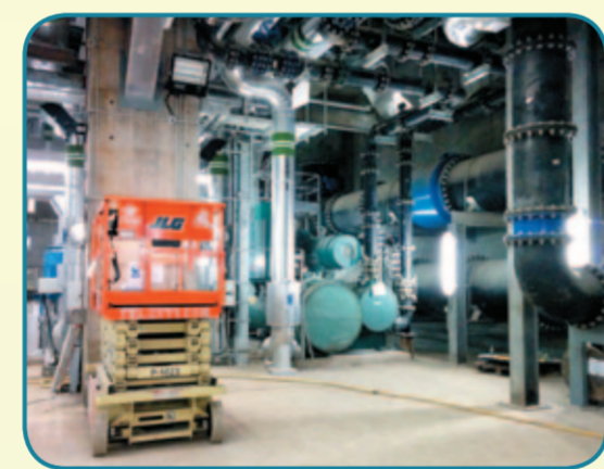
南廠制冷機組 South Plant Chillers
